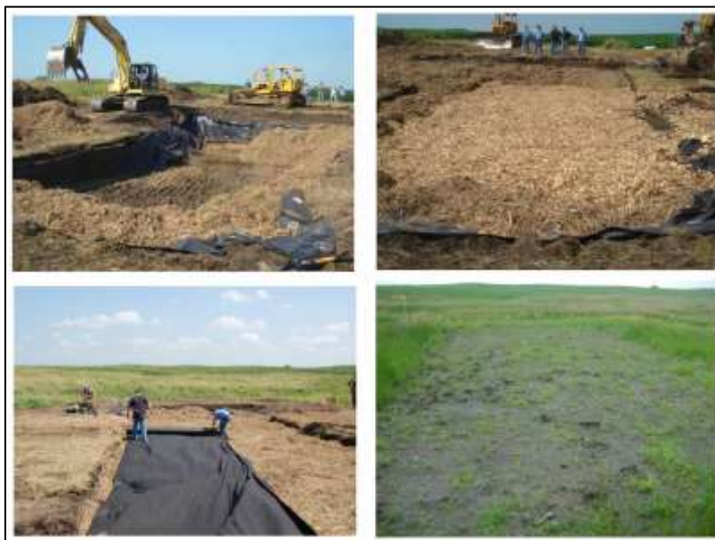
Bioreactor construction. (Ohio State University Extension)
